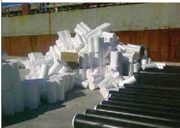
PLATE 40 Polystyrene cylinders are inserted into the pipes
